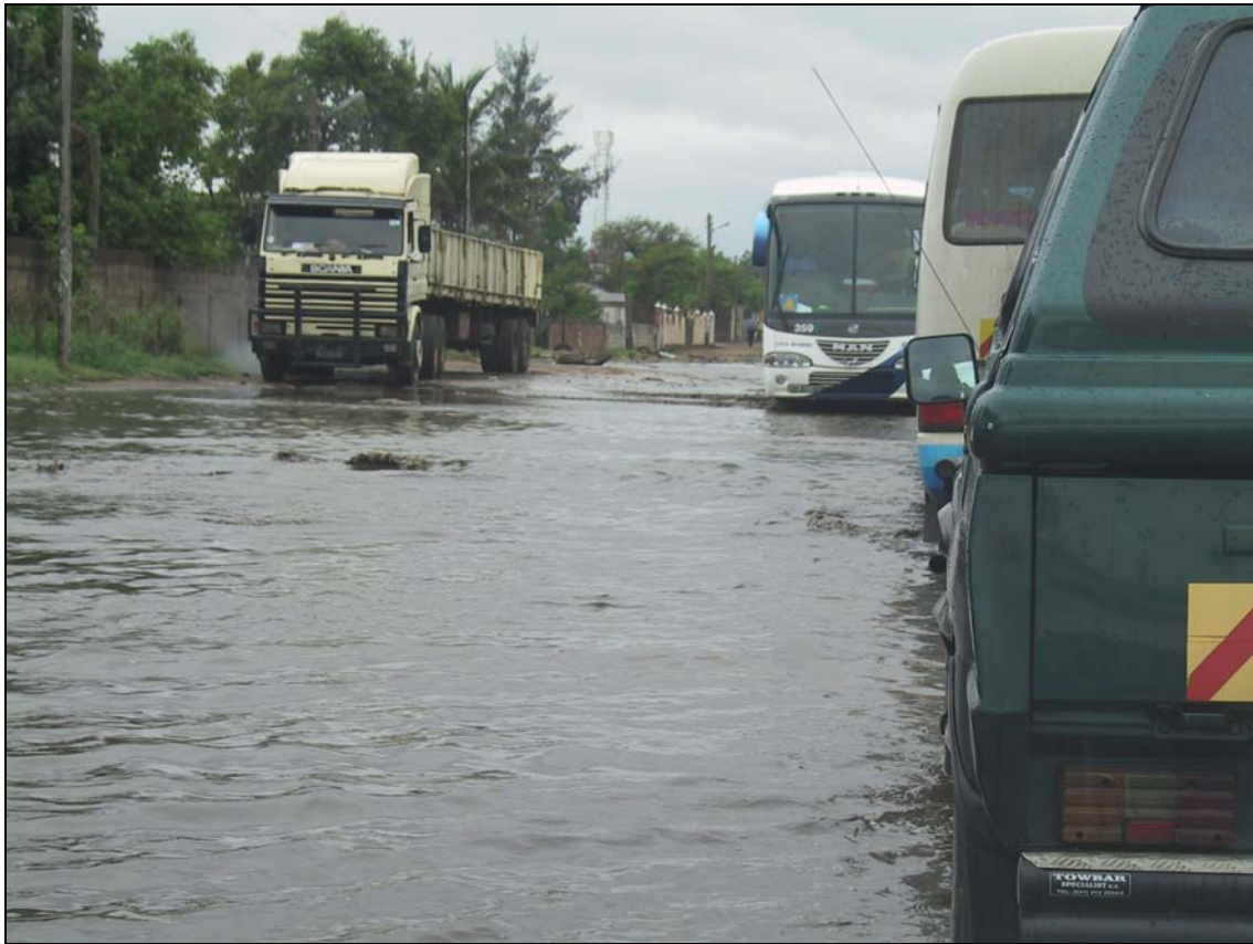
Figure 2-13: Lack of water drainage in Benfica causes traffic problems during rains.
